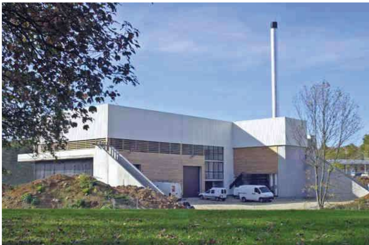
Chaufferie bois – Besançon – Doubs (25)
