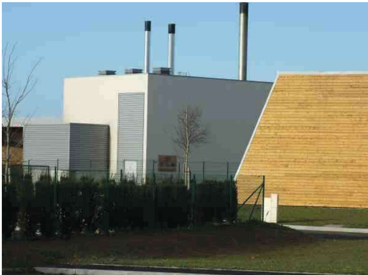
Chaufferie bois – Falaise – Calvados (14)
